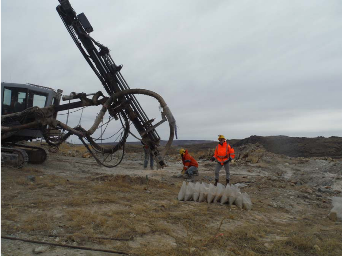
Figure 10.1.1. Rotary percussion drill (Eco Minera, Argentina contractor)
