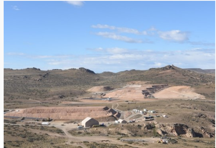
Lomada Project Site
