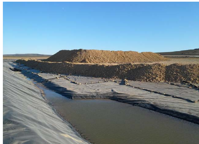
First ore loaded at Cap-Oeste HL Pad
