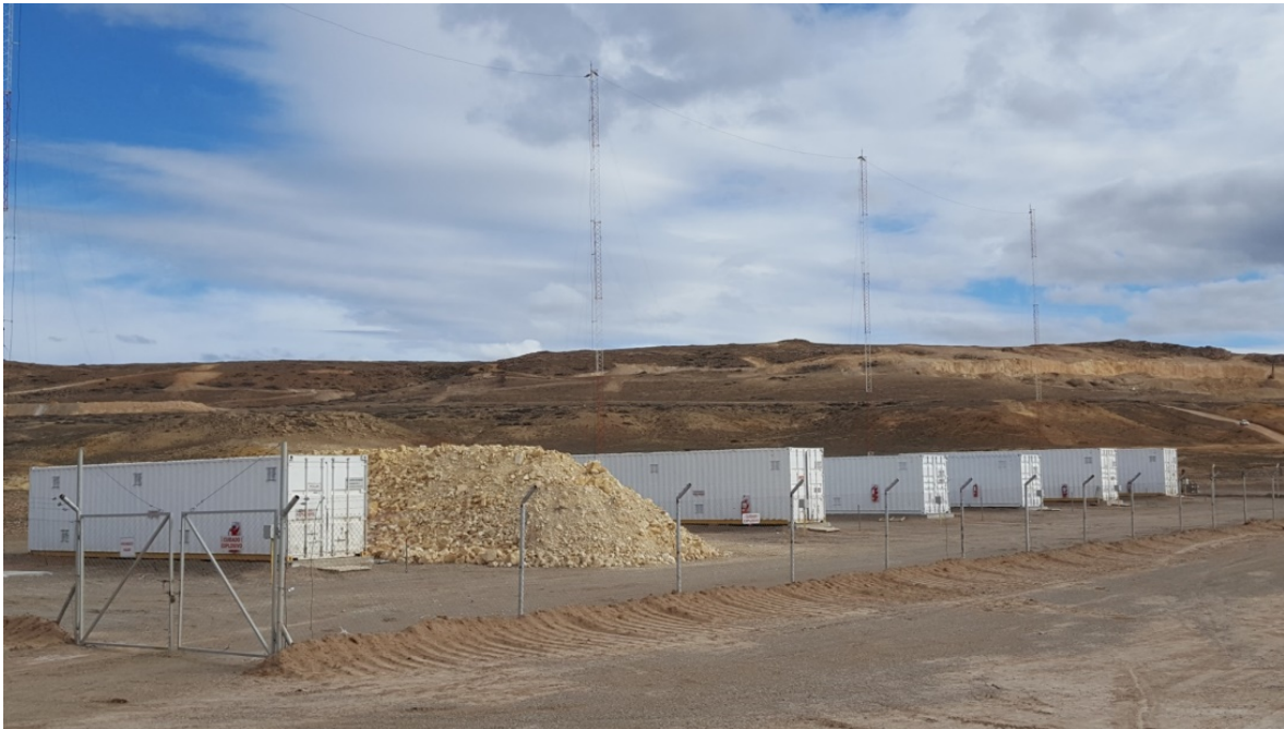
Completed blasting magazine at Cap-Oeste
