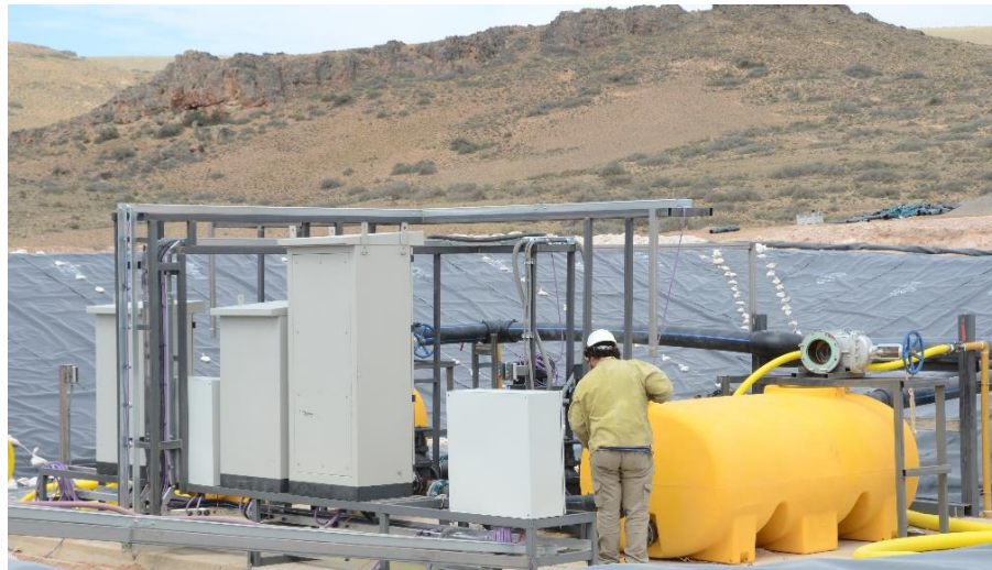
New Ponds and pumps commissioned
