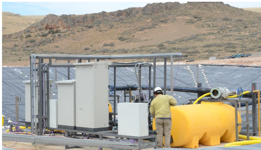
New Ponds and pumps commissioned
