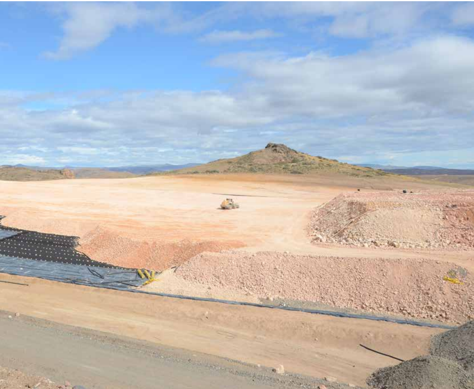
Loading of crushed filter material onto the Lomada pad
