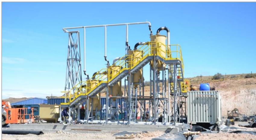
Construction of Plant Facility
