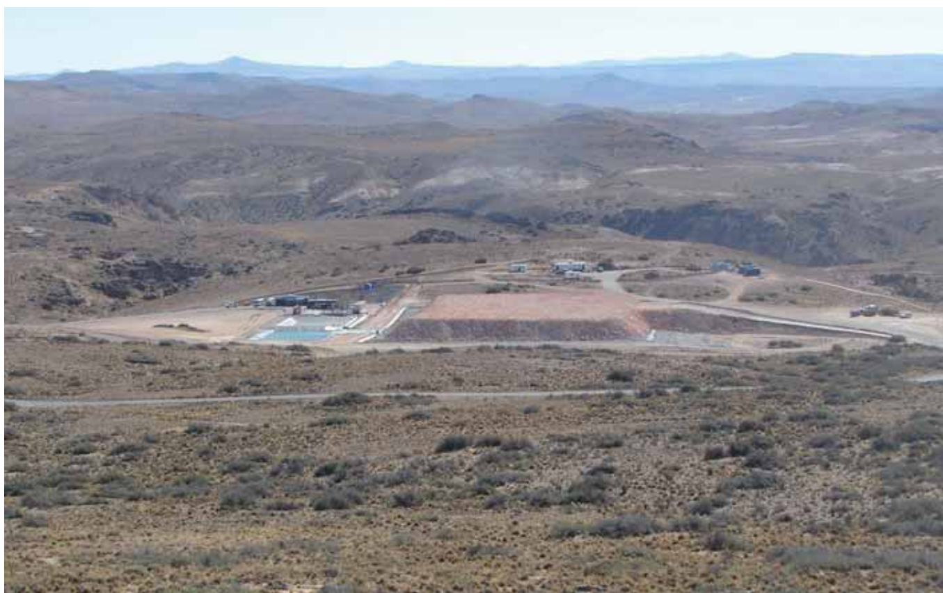
Lomada Trial Heap Leach Pad
