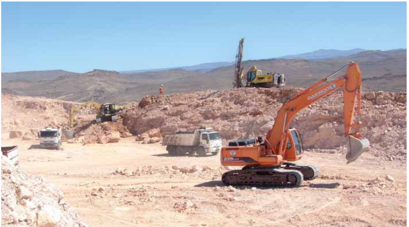
Lomada Mine Blast
